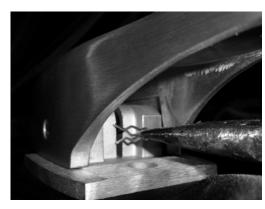
6. With door open, mount strike on jamb, lining up small boss with small hole. At the same time, push inside release rod through bask of inside jamb hole, through the wall until it engages threaded hold in back of strike.
