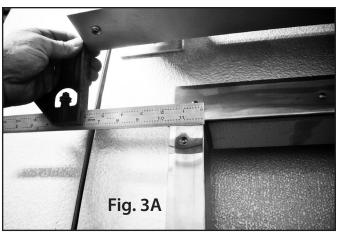
ets. Lift the rail, engage each pair of screw heads into the open slots in the mounting brackets. Then, at each Hanger Bracket, install the washers one at a time. At the closing side of the door, adjust the end of the rail so that it's 6" from door openings, as shown in the diagram (Fig. 3A). That will place the end of the rail ½" from the edge of that bracket. The door should stop such that the center of the roller is also at this 2 ½" from the end of the rail.
